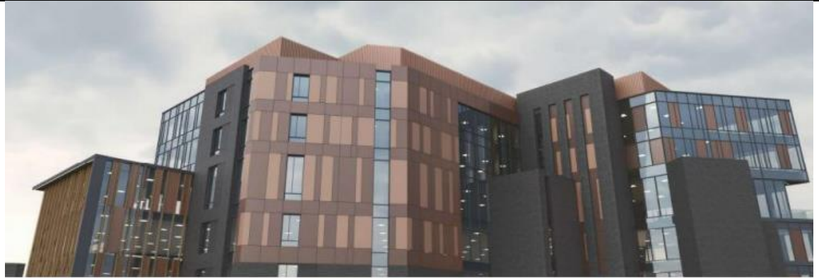
Figure 4: Rear of building
